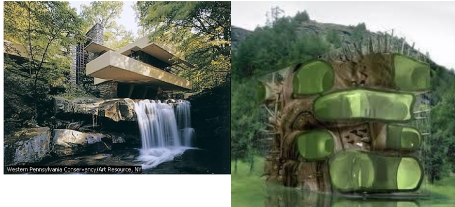
Fallingwater House. Fallingwater, the house designed by American architect Frank Lloyd Wright for the Kaufmann family, is cantilevered dramatically over a waterfall. The house was built of reinforced concrete and stone in the 1930s in Bear Run, near Pittsburgh, Pennsylvania, and appears to emerge from the landscape surrounding it. Western Pennsylvania Conservancy/Art Resource, NY. Microsoft® Encarta® 2009. © 1993-2008 Microsoft Corporation. All rights reserved.
