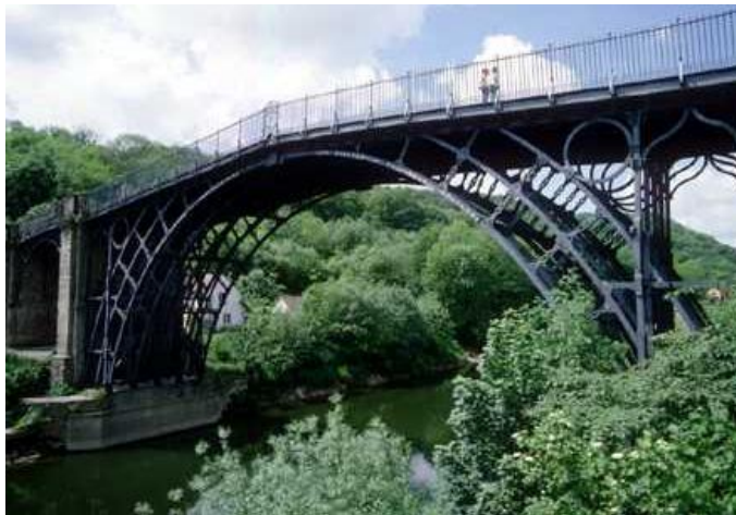
Ironbridge, Telford, England. Ironbridge, which crosses the River Severn in Telford, Shropshire, in western England, was completed in 1779. The first large-scale structure made of cast iron, the bridge was considered a remarkable feat of engineering at the time of its construction. Robert Harding Picture Library. Microsoft® Encarta® 2006. 1993-2005 Microsoft Corporation. All rights reserved.
